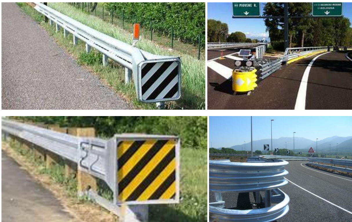
Figure 10 – Some examples of different safety elements protecting individual points.
