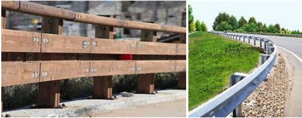
Figure 9 – Some examples of safety side barriers in different materials and with different characteristics.
